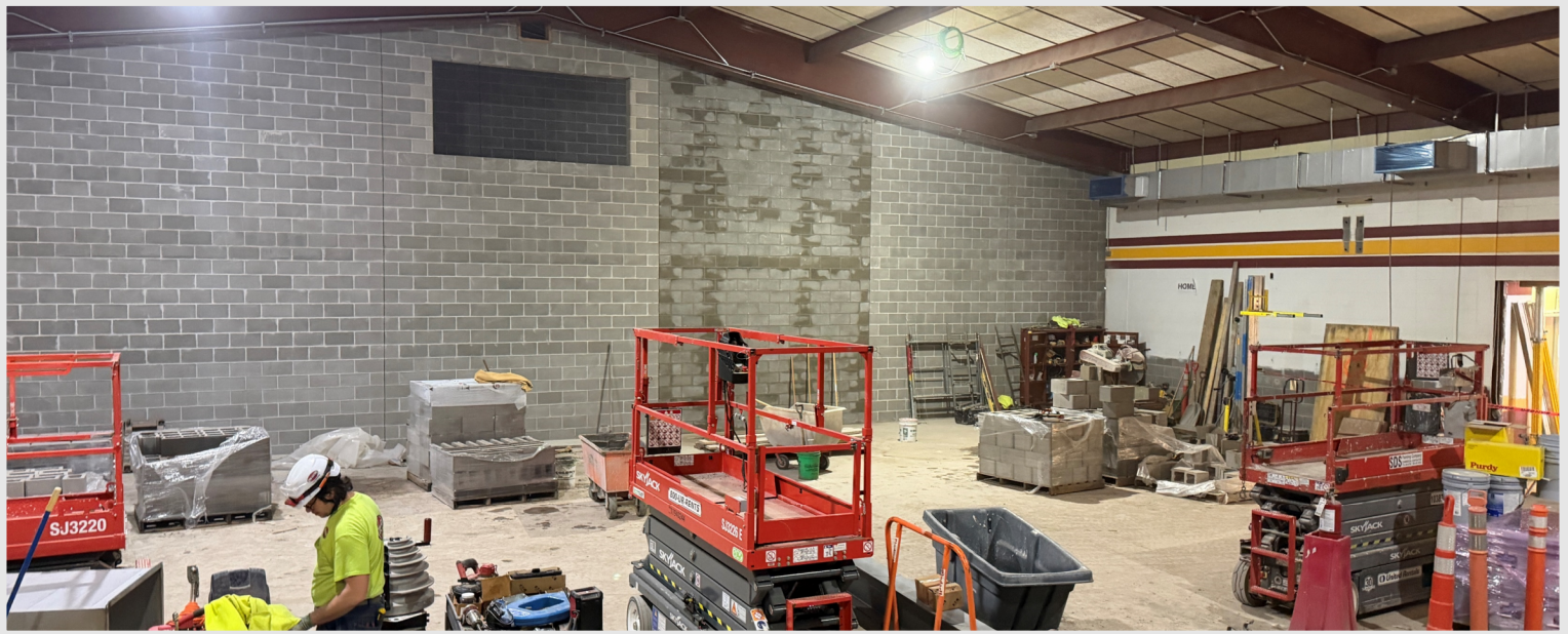
A view from the stage looking out towards the future cafeteria and new sound mezzanine.
