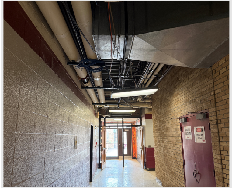
Existing ceiling tiles have been removed from the corridors outside of the band room to allow for mechanical piping installation.
