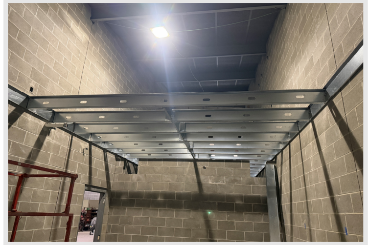
Framing has begun on the new sound mezzanine.
