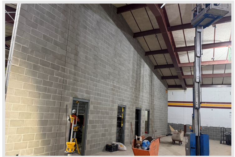
The wall separating the Band Room from the practice rooms has been constructed.
