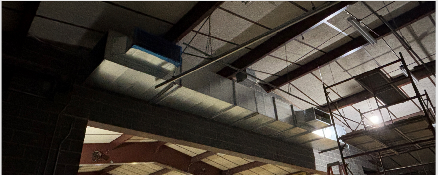
The new ductwork is getting installed above the stage.
