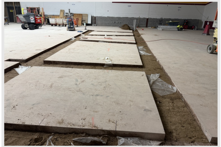
Phase 3 Demolition Progress
