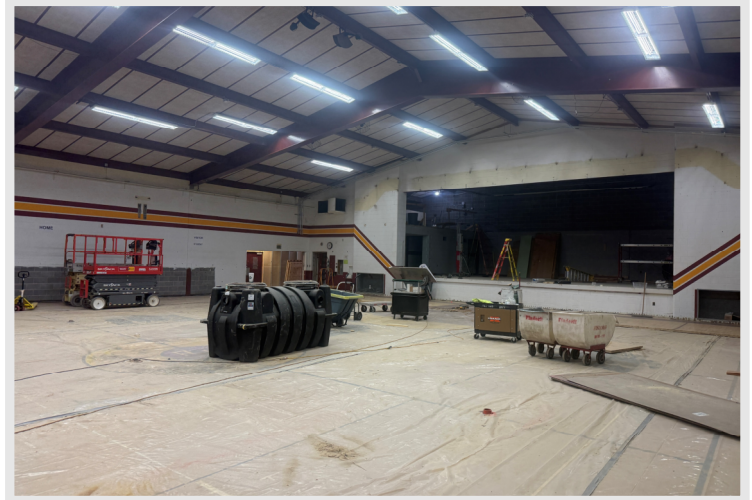
Phase 3 Demolition Progress
