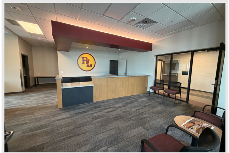
The completed reception desk is ready for the staff to move in.
