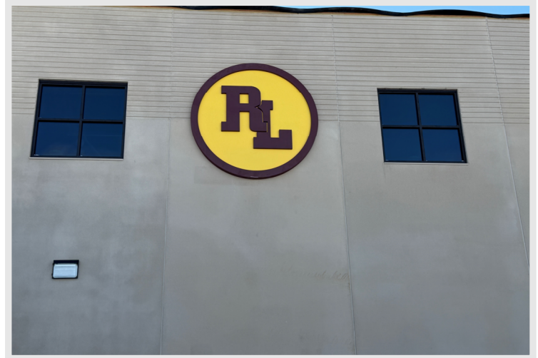
The exterior signage on the gymnasium has been installed.
