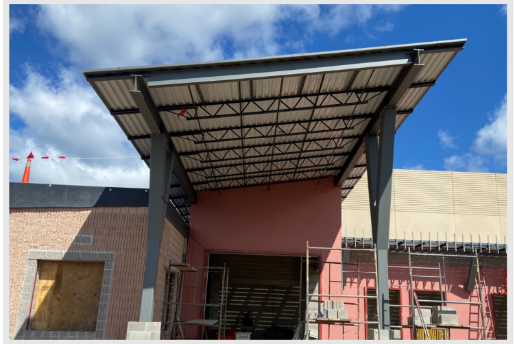
The canopy over the new main entrance has been installed and awaits the completed brick around the columns.
