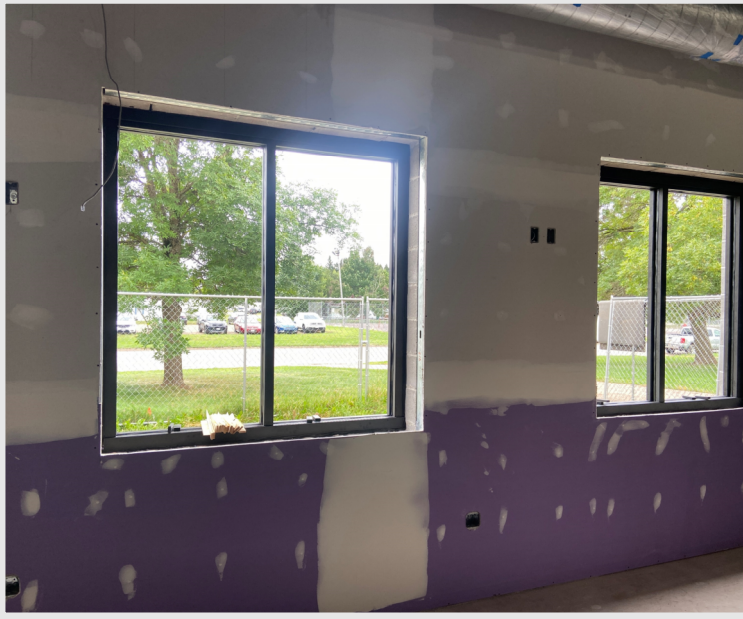
The aluminum frames for the new fitness room have been installed and await the glass installation.
