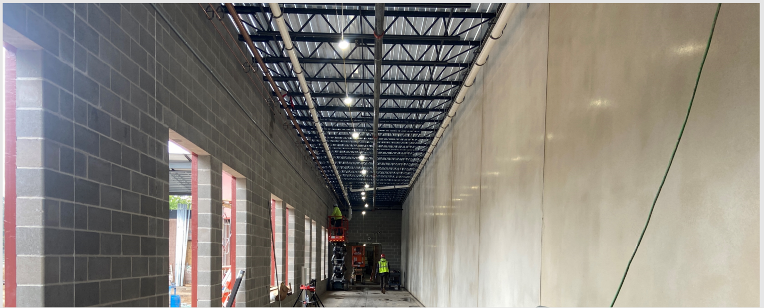
The overhead plumbing and fire protection installation has begun in the addition corridor.
