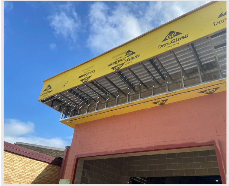
The exterior framing has been completed around the north vestibule and is now ready for spray foam.
