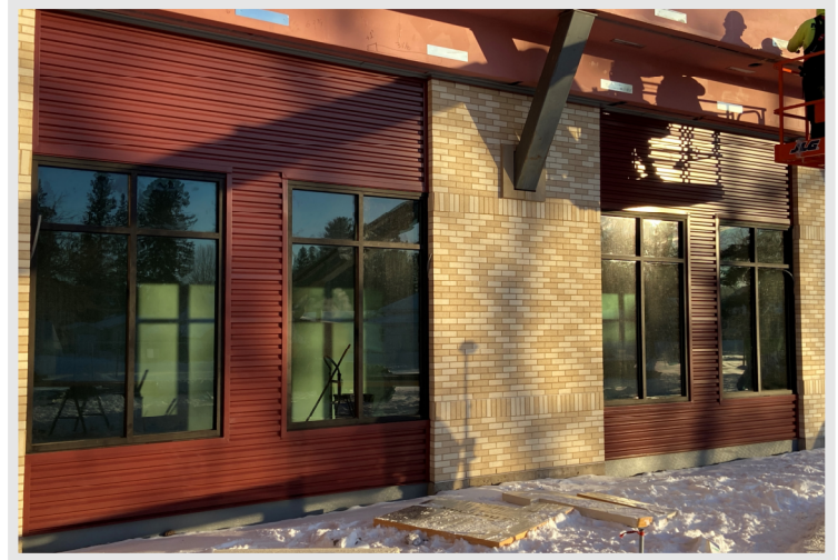
Metal panel installation has continued with the corrugated panel wrapping up.
