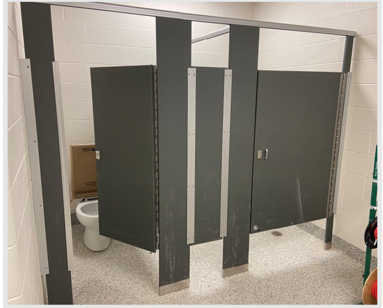
The bathroom partitions have been installed in the addition restrooms.
