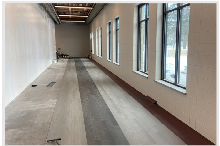
The luxury vinyl tile installation has begun in the south corridor.
