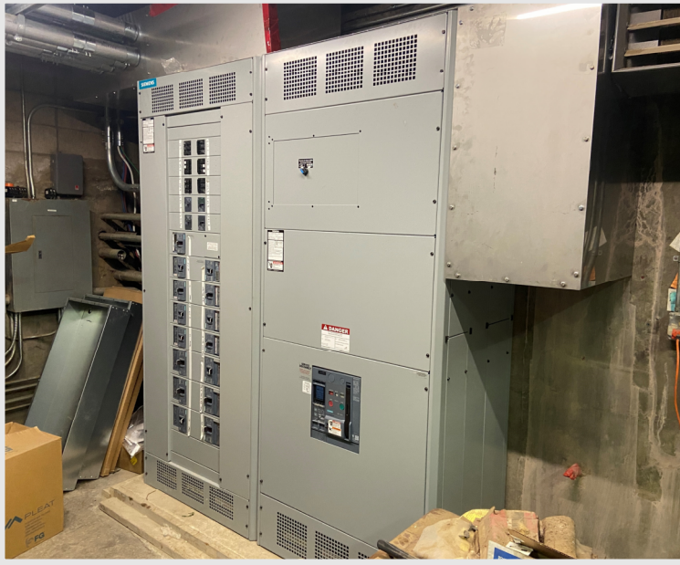
The new switchgear has been installed inside the boiler room after a successful shut down.
