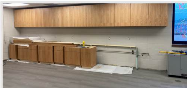
The flooring and ceiling have been installed inside of the newly renovated middle school science room. Up next is to finish setting the base cabinets.
