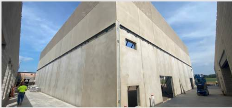
The precast panels for the new gym addition have been set, allowing us to start installing the roof joists and decking.
