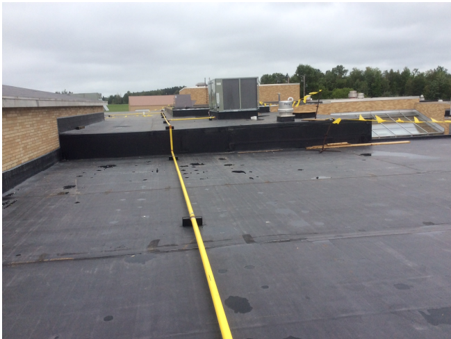
A section of completed roof at the High School.
