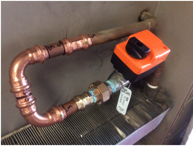
New digital controls are being installed on existing equipment.
