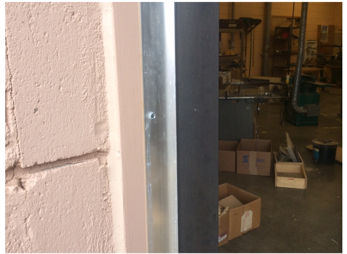
Weatherstripping has been installed on doors improving overall building performance.
