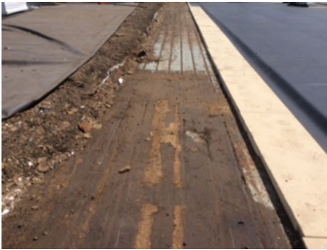
Old roofing systems have been removed down to the metal deck.
